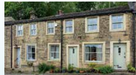
Historic building retrofit
