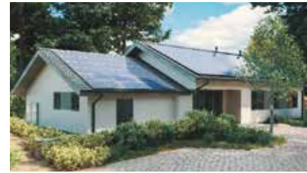
Deep energy retrofit
